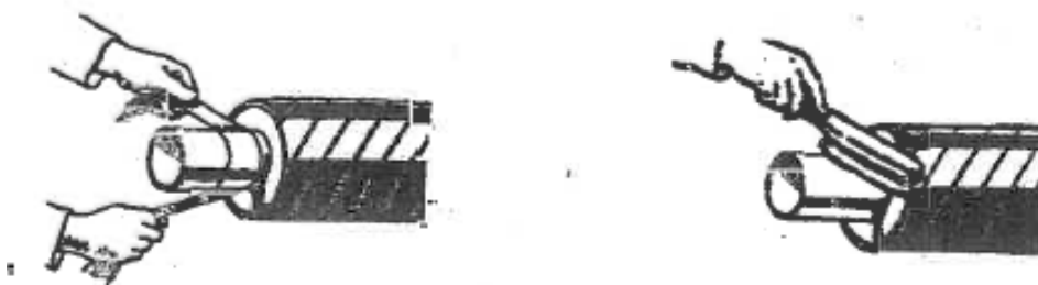
Preparation of service and casing pipe surface prior to application of heat-shrink sleeve.
