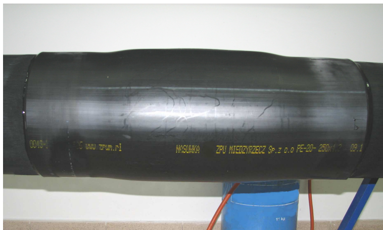
Photo No. 30 View of radiational crosslinked heat shrinkable sleeves after shrinking.
