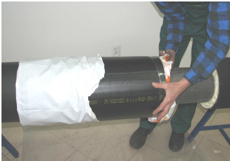
Photo No. 25 Removal of white foil from radiational crosslinked heat shrink sleeve
