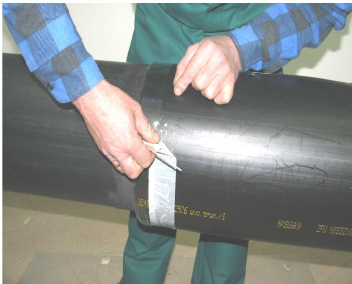
Photo No. 26 Removal of inner foil protecting the glue in radiational crosslinked heat shrink sleeve.
