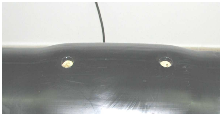
Photo No. 44 Purification of the filling holes of welded plugs mounting places
