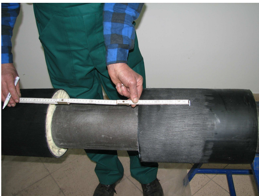
Photo No 24 Designation of calculated dimensions at determining the position of the edge of the radiational crosslinked heat shrinkable sleeve
