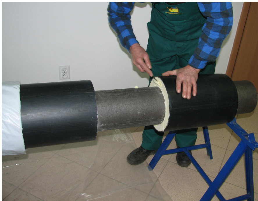
Photo No. 21 Remove with a knife or scraper, the thermal insulation - PUR foam with a thickness up to 15 mm from the face of preinsulated bonded parts.
