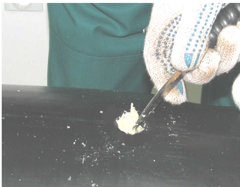
Photo No. 42 Removal of the PUR foam from filling holes to a depth of about 5 mm
