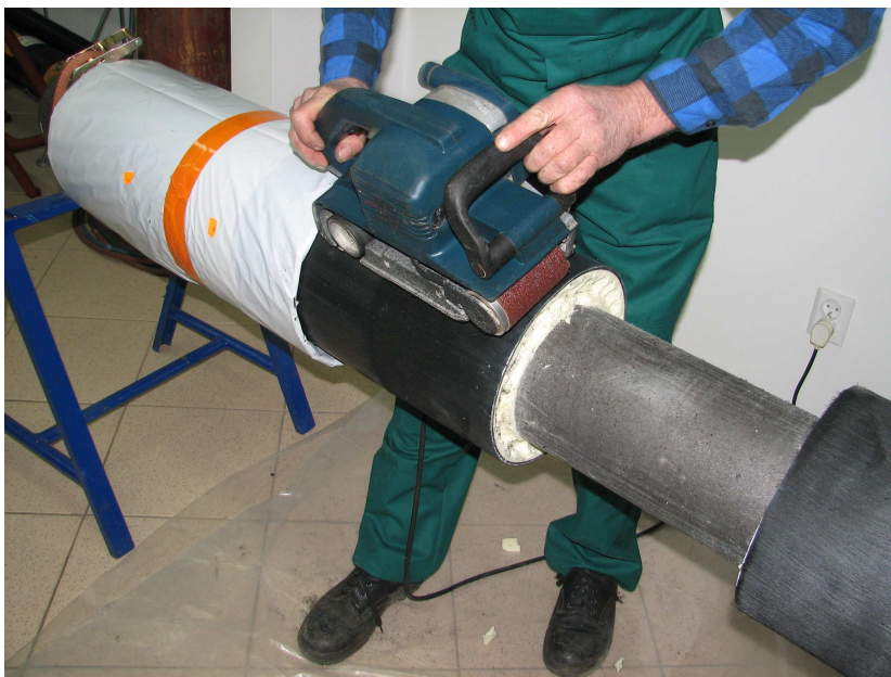
Photo No. 22 Cleaning the casing pipe of preinsulated element using a belt grinder with sandpaper grit 50 \pm 70
