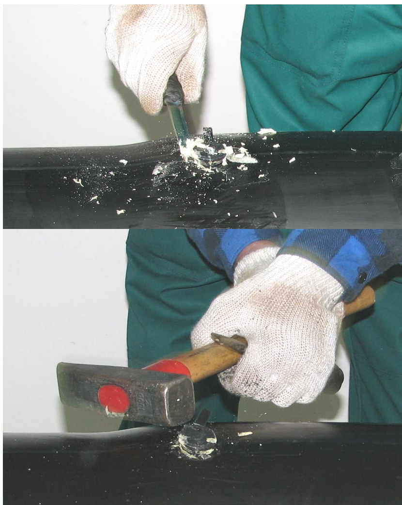
Photos Nos. 40 and 41 Removing the vent plugs from the filling holes
