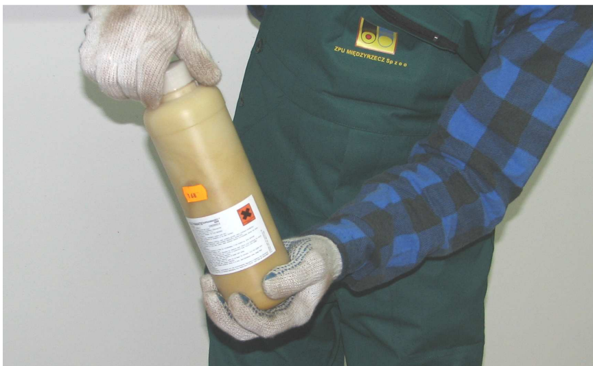
Photo No. 36 Mixing of PUR foam components A and B
